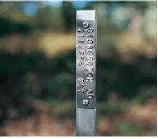
Marking of site boundaries with tags of stainless steel or aluminum is a durable solution.
