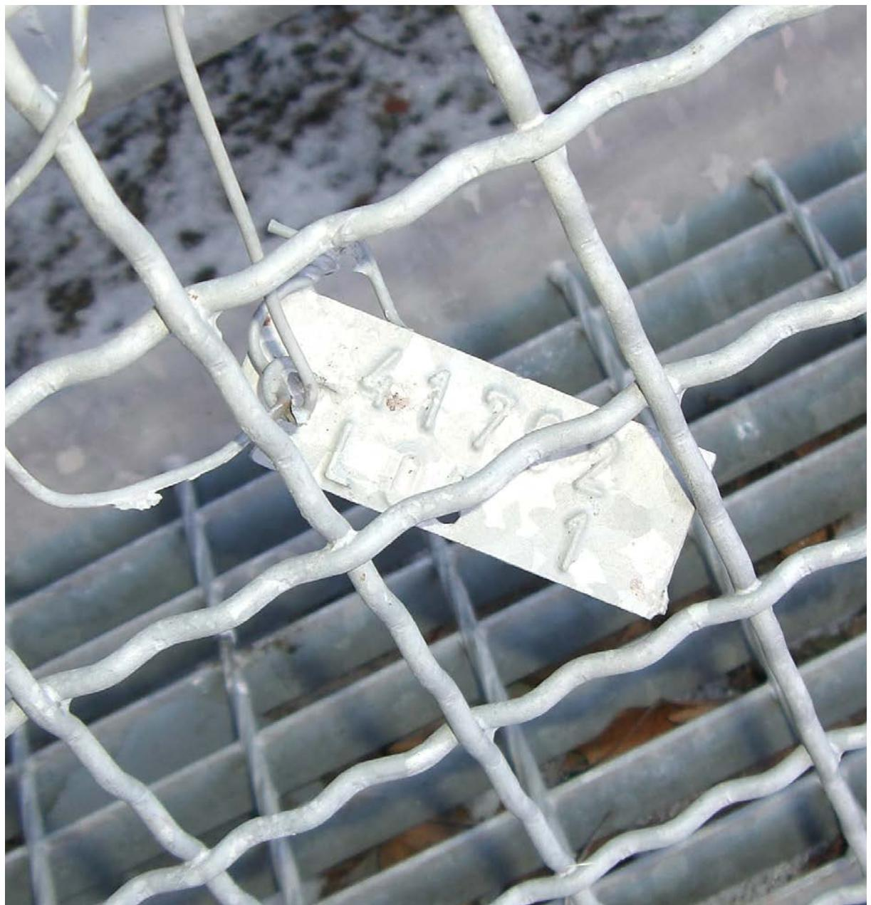
Weland die sunk marking tags can be made of hot-dip galvanized steel metal or stainless steel. Manufactured in single-row or two-row versions.
